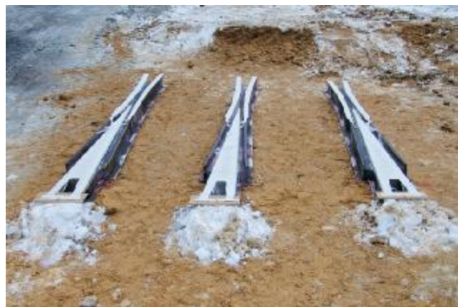
Application of the sheet explosive during railway frogs explosive hardening
